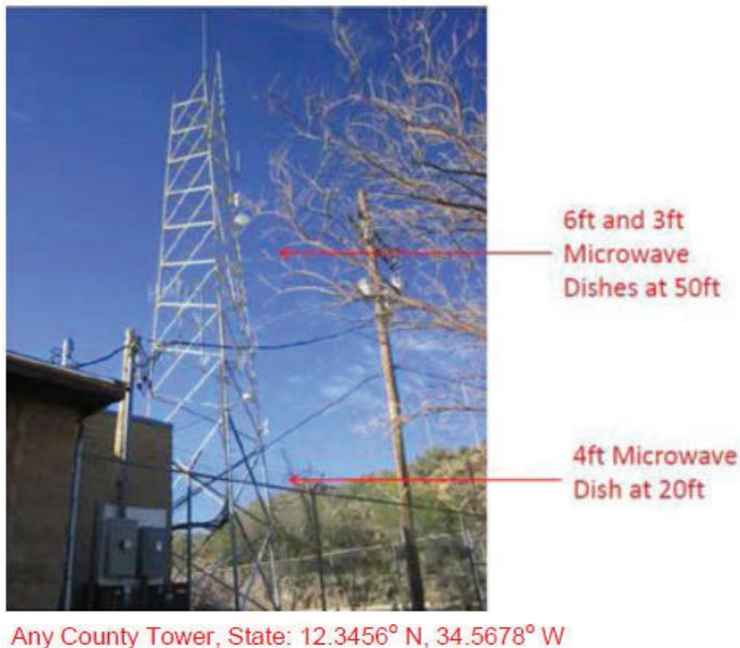
Any County Tower, State: 12.3456° N, 34.5678° W Figure 5. Ground-level photograph showing proposed locations of new communications equipment on an existing tower.
