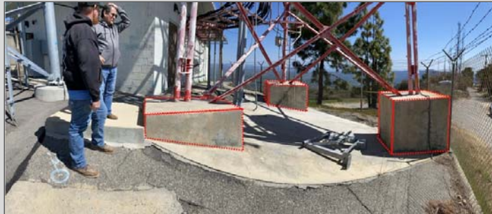
Photos of CPK Tower
